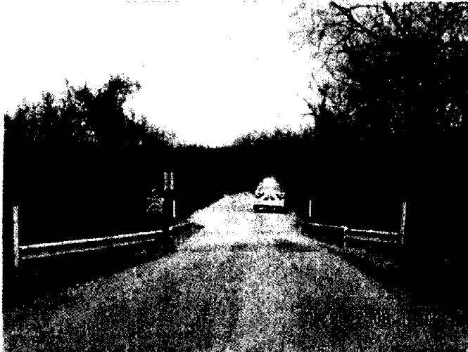
02-249-AA02-05-002 SLZ 1/28/2008 CR 2560 over Branch of Denton Creek Approach looking NW with Load Posting signs.
